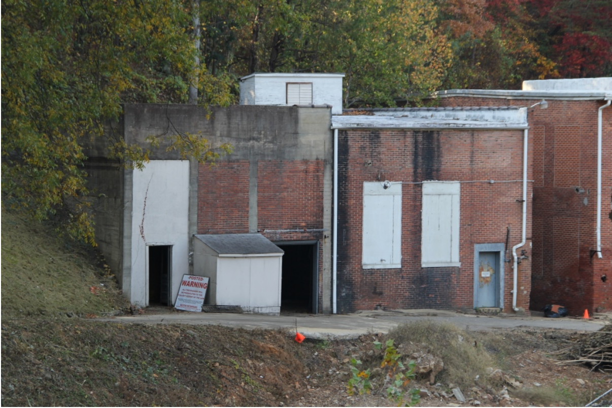
South end of the east wing of Tryon Hosiery Mill, view to northwest
