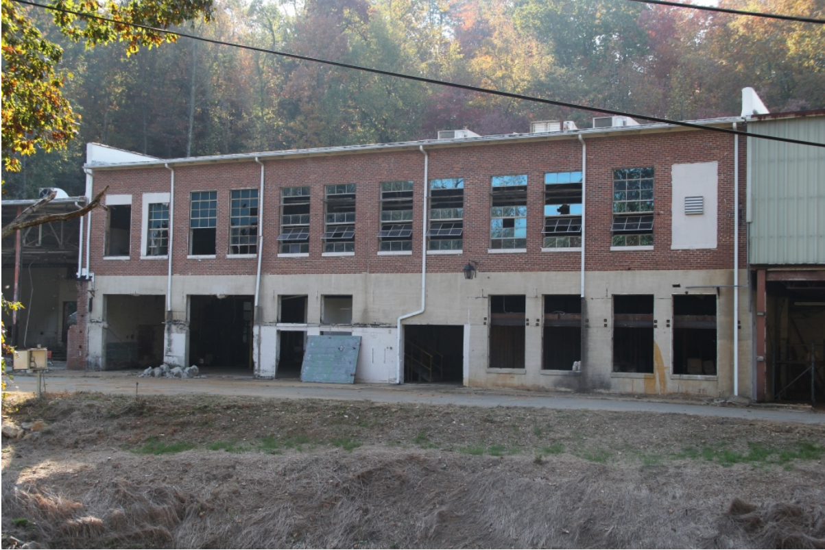
East wing of Tryon Hosiery Mill, view to west
