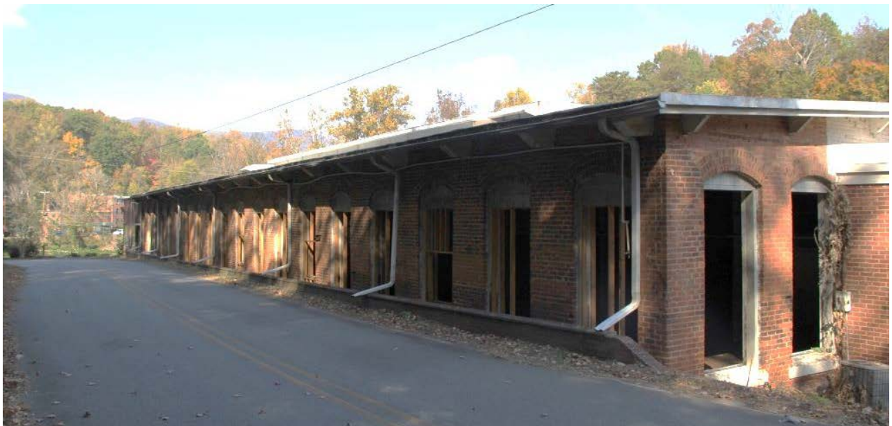
Tryon Hosiery Mill, west elevation, view to north along Clarence Rhodes Road
