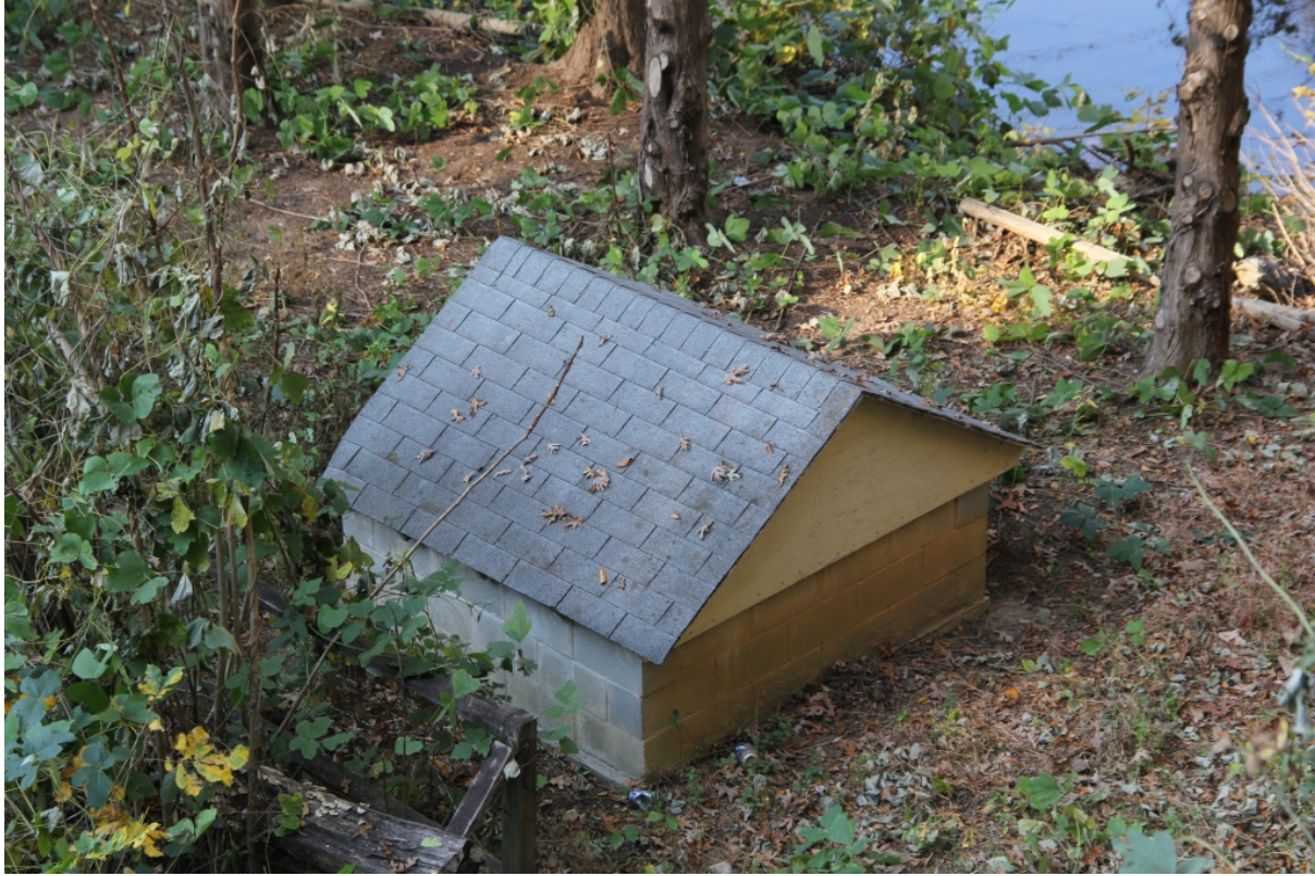
Pump house, Tryon Hosiery Mill, view to north
