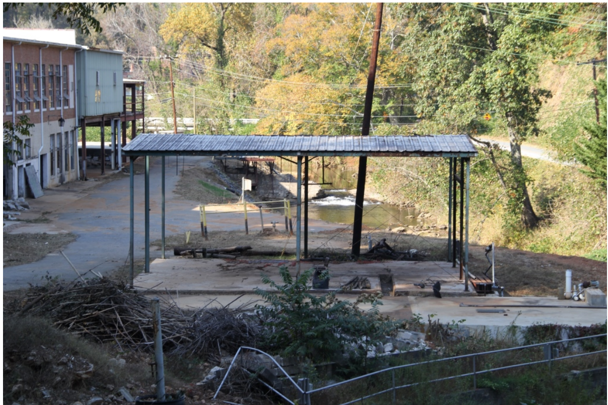
Shed, Tryon Hosiery Mill, view to north
