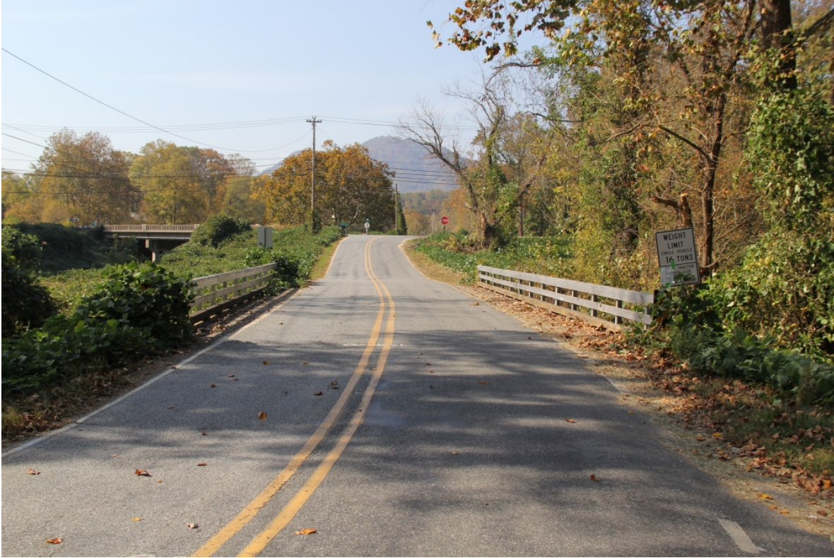
Bridge No. 63, view to northwest along SR 1543 (Capps Road)
