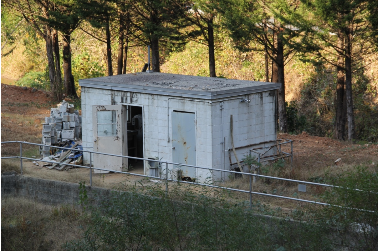
Maintenance building, Tryon Hosiery Mill, view to northeast
