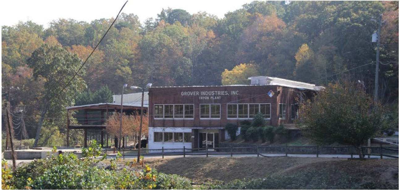
Tryon Hosiery Mill, façade, view to south from NC 108 (Lynn Road)
