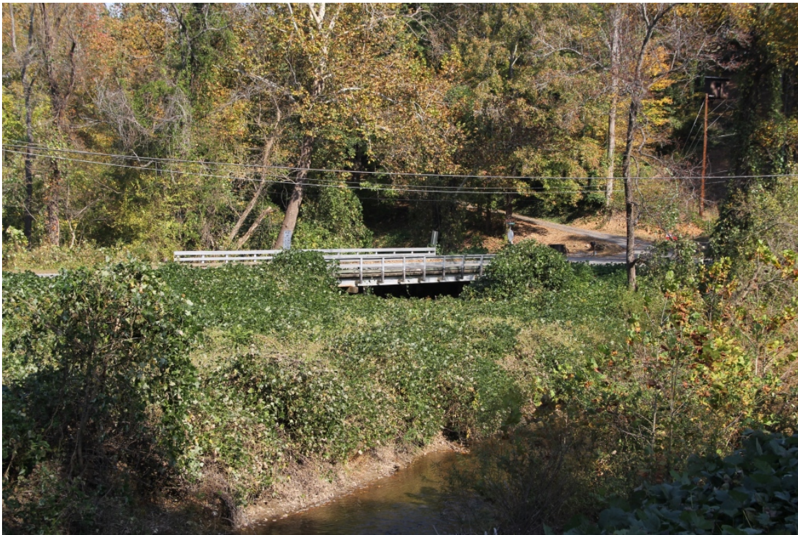
Bridge No. 63, view to southeast from NC 108 (Lynn Road)
