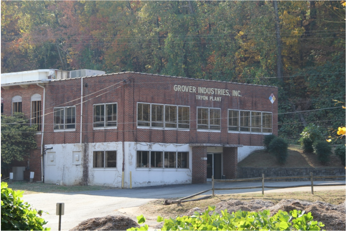
Office wing, Tryon Hosiery Mill, oblique view to southwest
