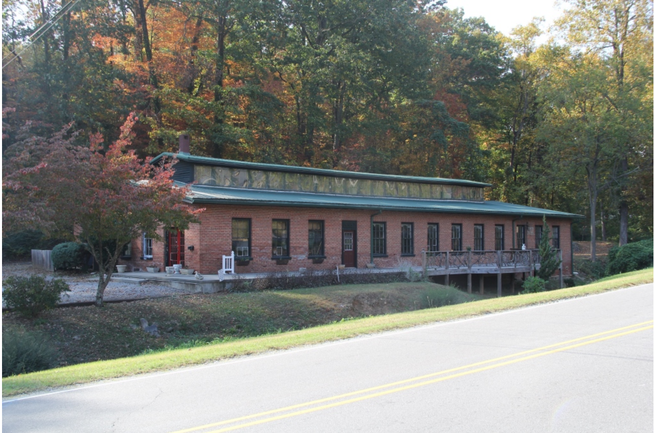
Tryon Hand Weavers Building (PL 298), ca. 1940, oblique view to west
