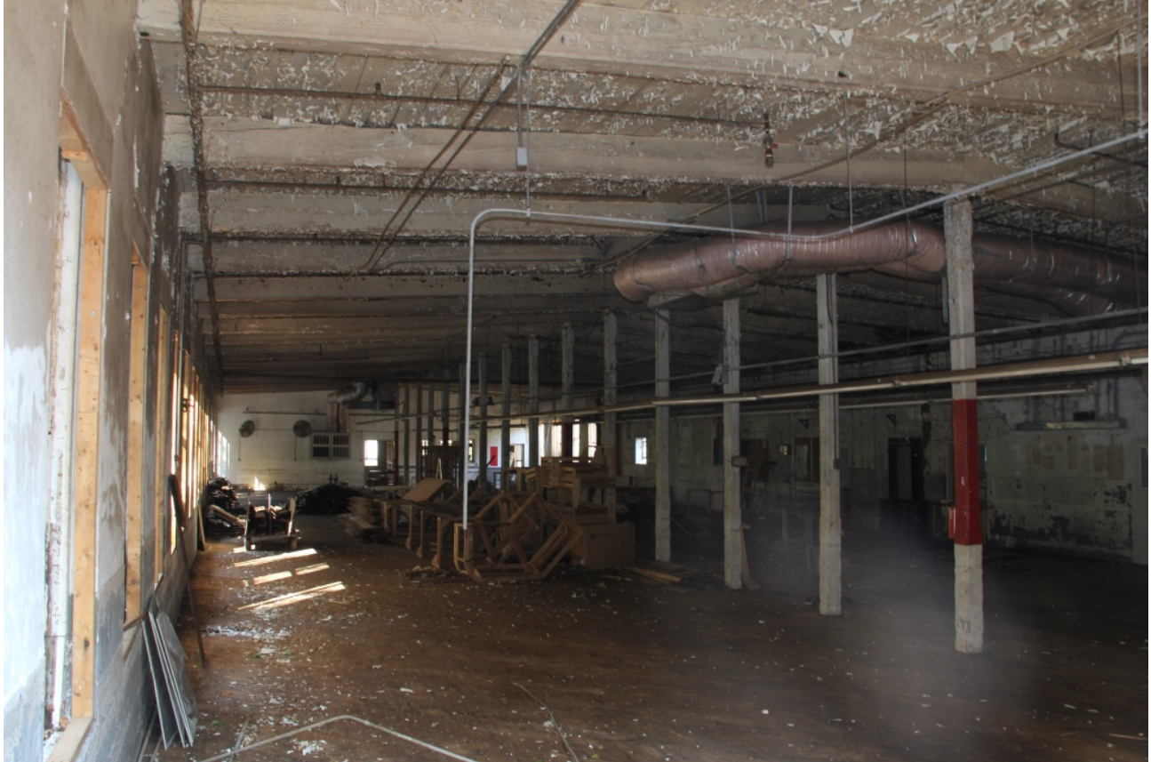
Main mill floor, interior, view to north
