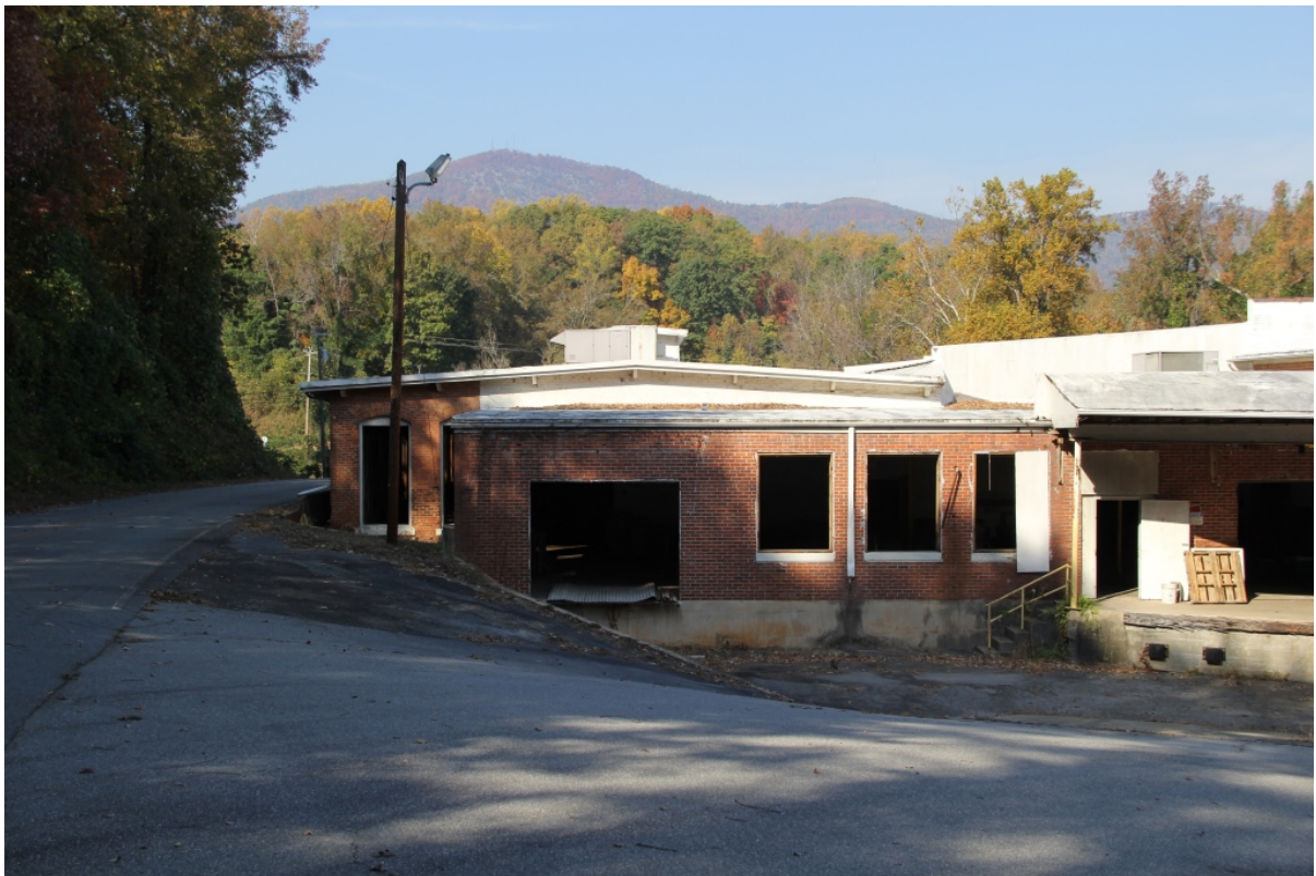
Distribution wing, Tryon Hosiery Mill, view to north
