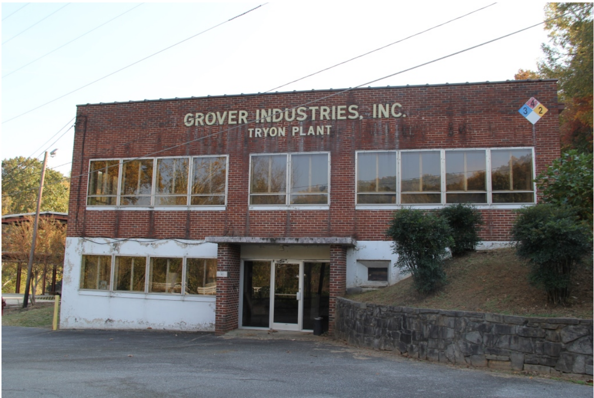
Office wing, façade, Tryon Hosiery Mill, view to south
